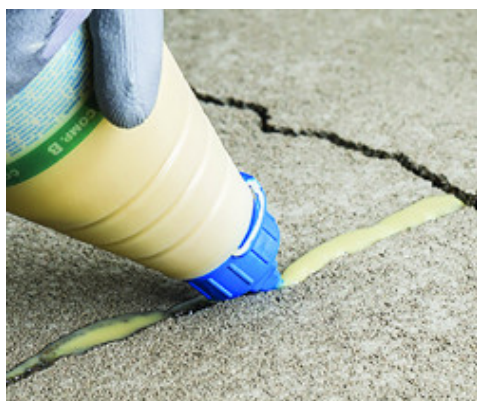
Pour the product into the crack using the nozzle
