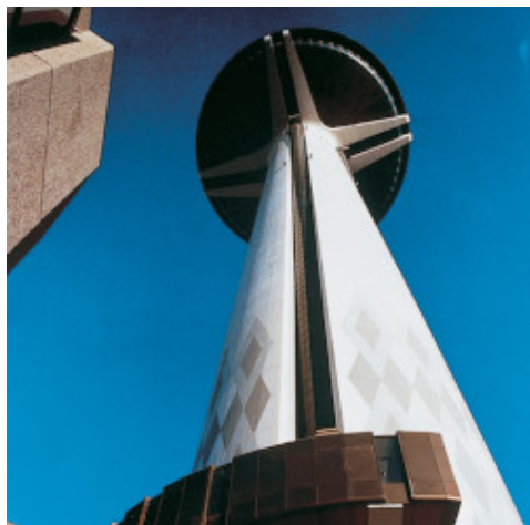
An example of an installation of klinker on concrete with Kerabond + Isolastic - New Telecommunication Tower - Kuwait City (Kuwait)
