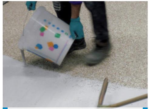
Application of Ultratop on the hardened surface of the mixture made of natural aggregates + Mapefloor 910
