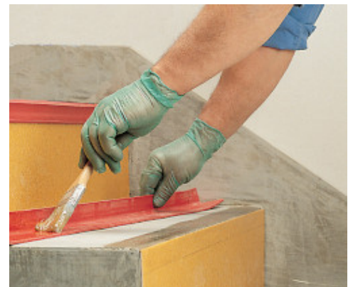
PVC installation on a step
