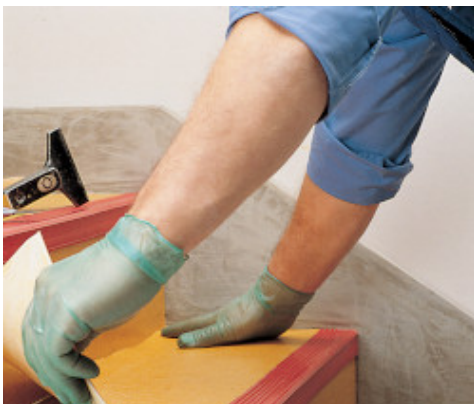
Spreading Adesilex VZ of the backing of a PVC covering
