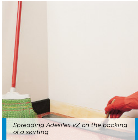
Bonding of PVC skirtings
