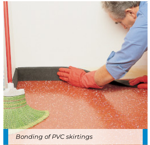
Spreading Adesilex VZ on the backing of a skirting
