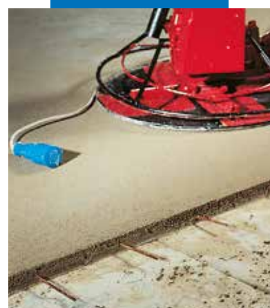
Power floating the surface of a Topcem screed
