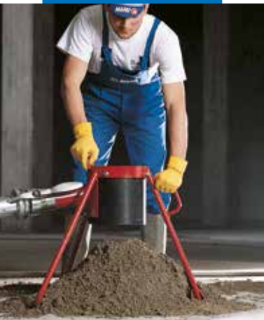
Batching a Topcem mix
