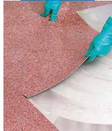
Installing PVC with Adesilex G19
