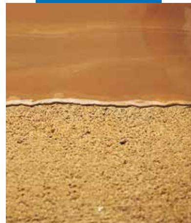
Finishing a Mapecem screed with Ultraplan Eco self-levelling compound
