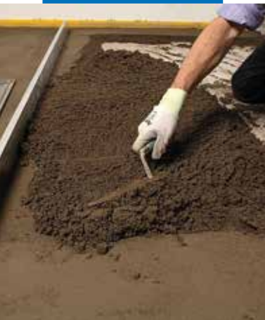
Applying and levelling the screed
