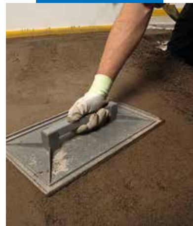
Compacting the screed
