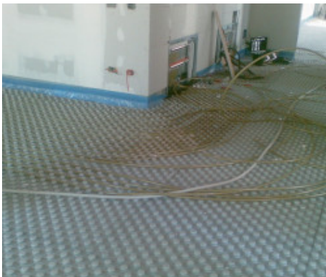
Preparation of the heating/cooling system
