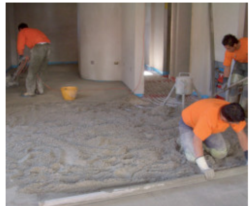
Spreading the mix with Mapescreed 704 admix
